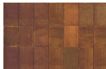
Fasad Weathering Steel (Corten Stål)
